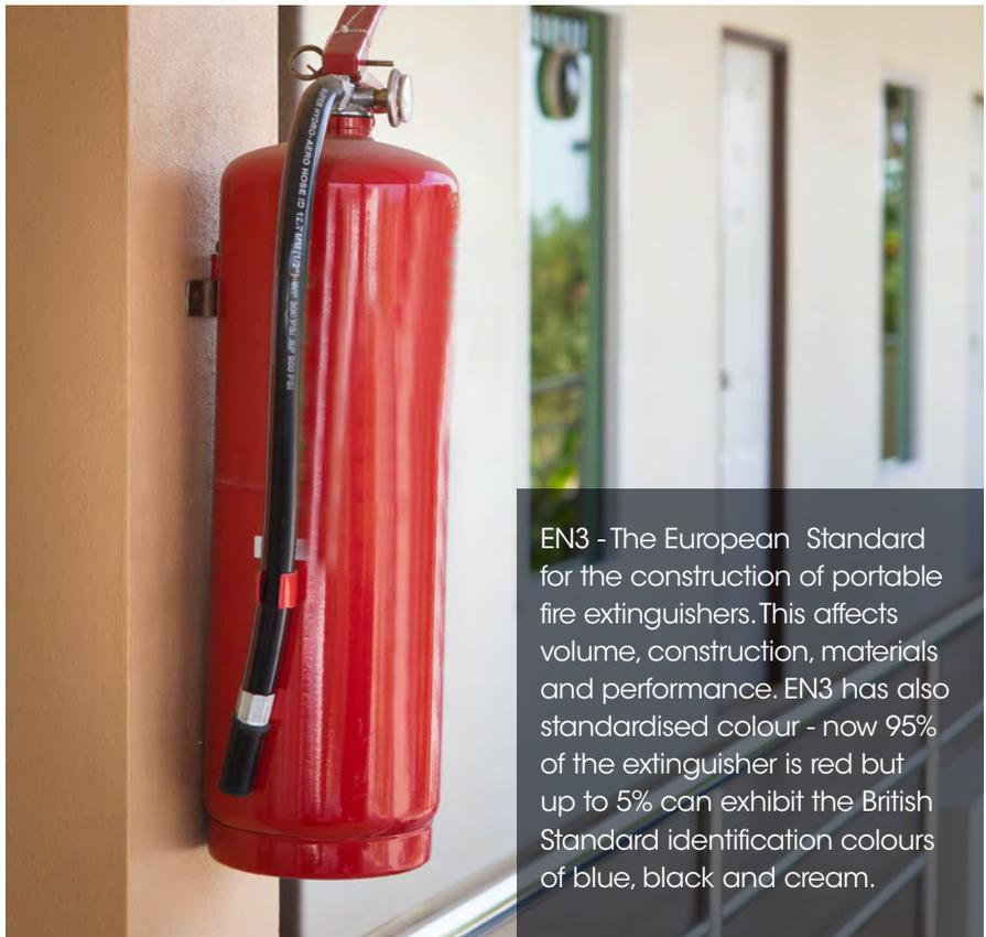
EN3 - The European Standard for the construction of portable fire extinguishers. This affects volume, construction, materials and performance. EN3 has also standardised colour - now 95% of the extinguisher is red but up to 5% can exhibit the British Standard identification colours of blue, black and cream.
